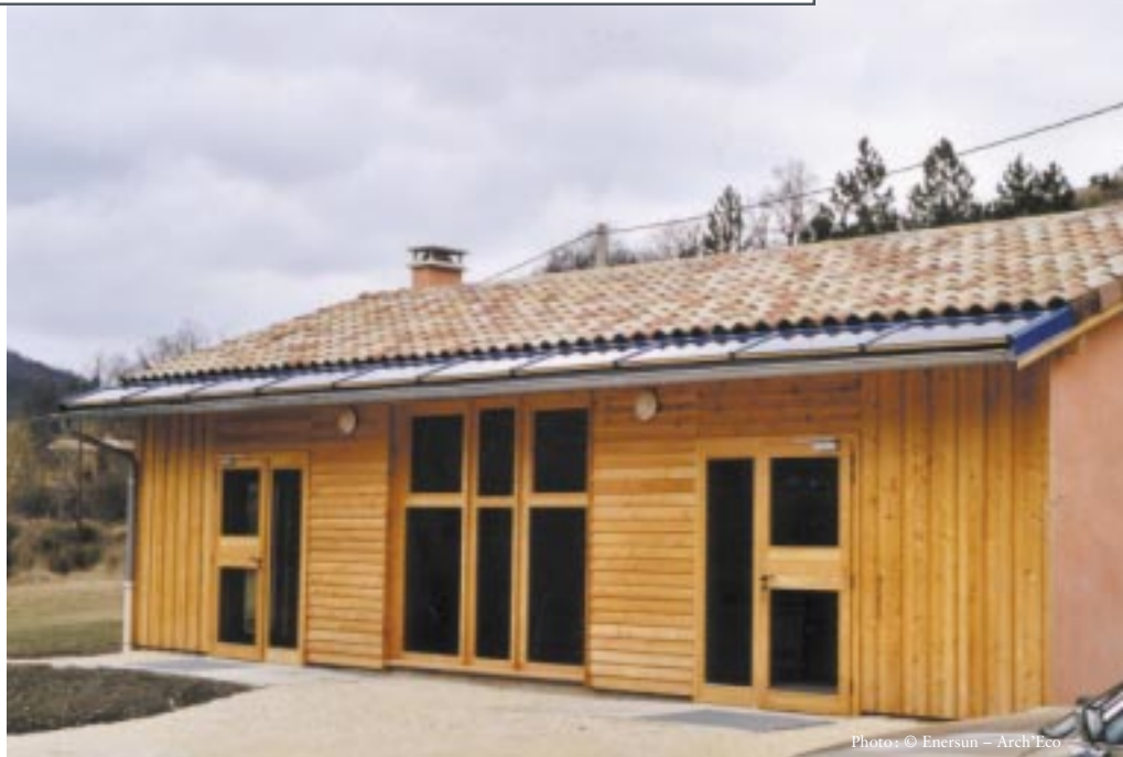
Photos © Enersun - Arch'Eco
